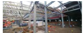
Fig 9.7 Steel Frame During Construction
