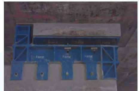
Fig 5.4 Farrat 2,000 kN Column Head Shear Key For Offset / Walking Column
