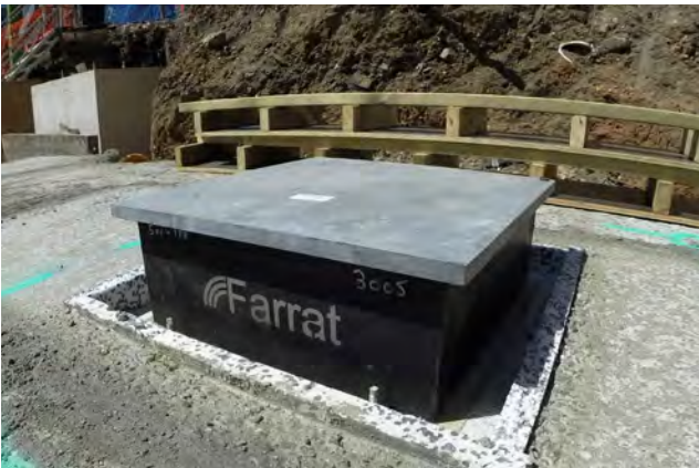
Fig 10.4 Farrat Natural Rubber Laminated Acoustic Bearing
