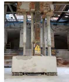
Fig 9.4 Isolation of Retained Façade
