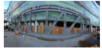
Fig 9.6 Large Truss Supported by Farrat Isolation Bearings
