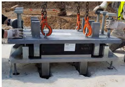
Fig 5.3 Farrat 700 kN Shear Key Unit Being Installed Into Pile Cap
