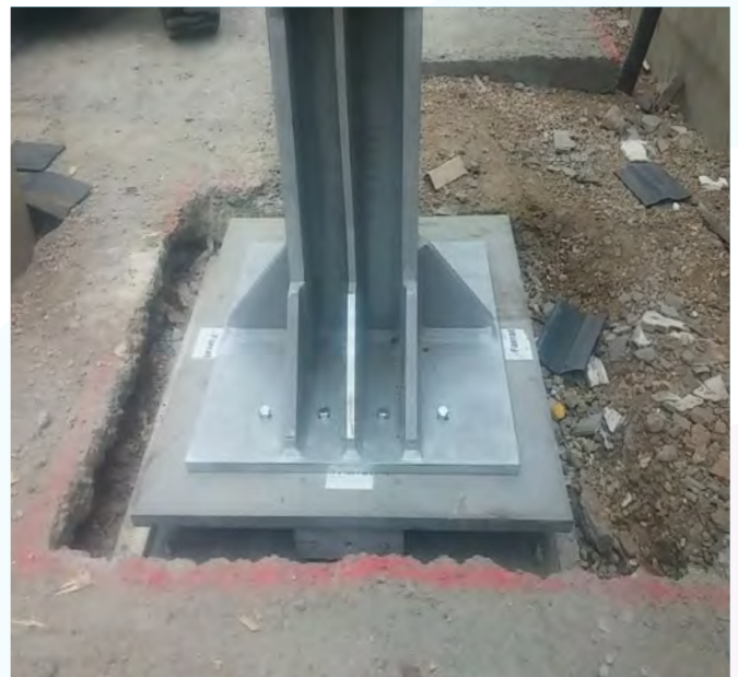
Fig 10.6 Bearing Assembly Supporting an External V Column
