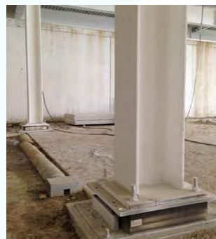
Fig 3.3 & Fig 3.4 Farrat LNR Bearings Supporting Steel Frames
