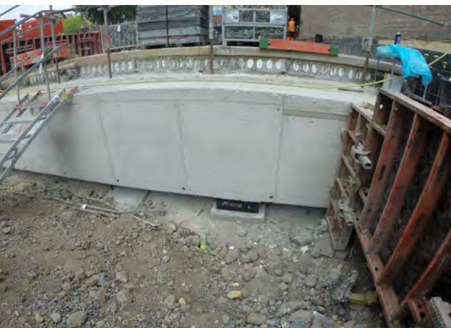
Fig 10.5 Farrat Natural Rubber Laminated Acoustic Bearing
