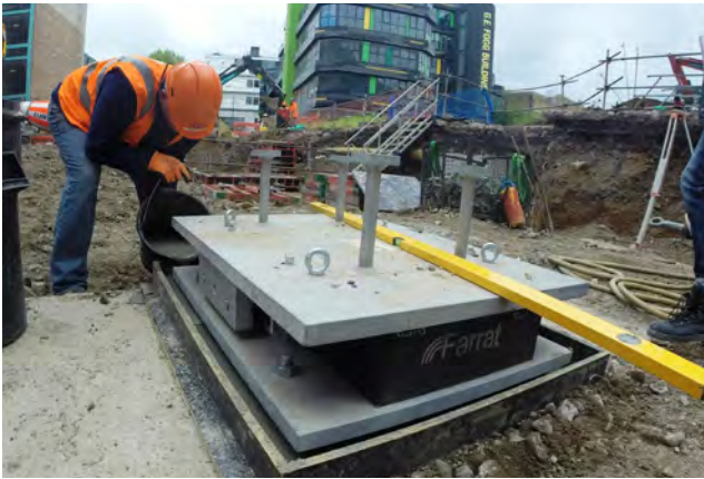
Fig 10.3 The Lateral Restraint Bearing Assembly During Installation
