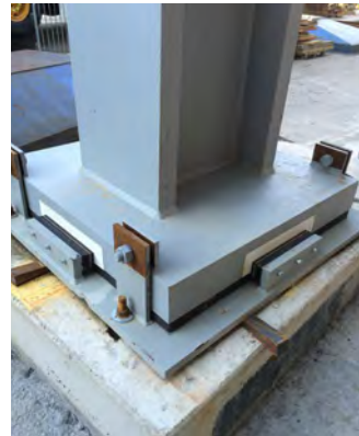
Fig 9.5 Isolation Bearing Assembly With Temporary Construction Restraints
