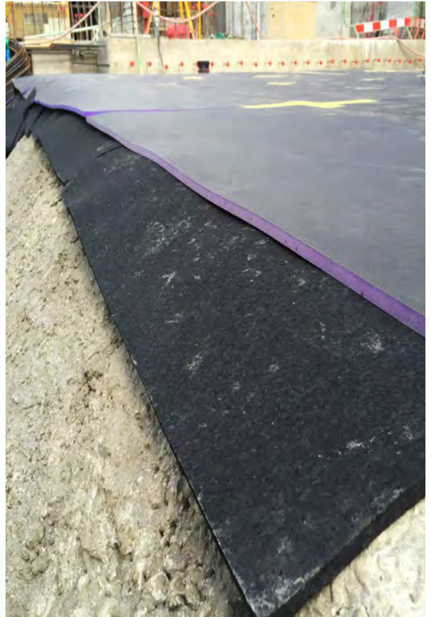
Fig 10.10 Farrat Full-Area Isolation mat
