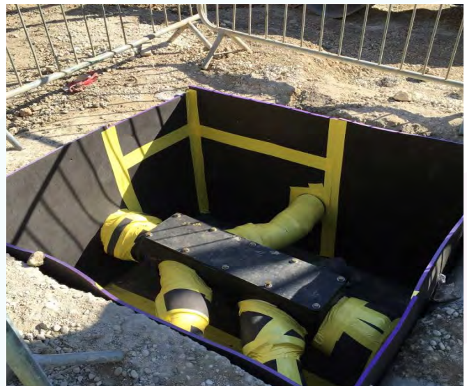
Fig 10.9 Isolation Detailing of Services
