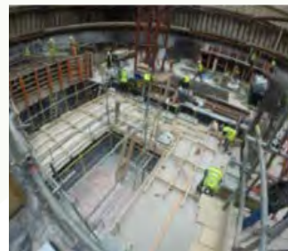
Fig 9.3 Construction of Cores
