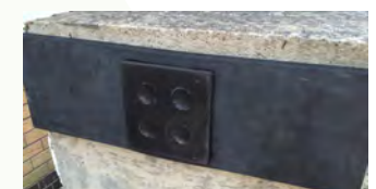
Fig 5.12 Lateral Restraint Bearing Within ISOFOAM Pocket
