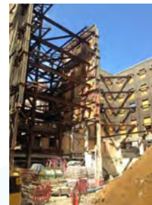
Fig 6.5 Retained Façade
